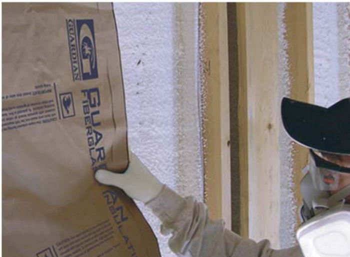
Application of kraft faced or unfaced fiberglass insulation; depending on Climate Zone.
