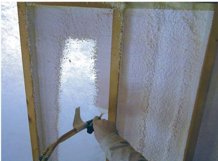
Spraying closed-cell foam against polyester mesh on open wall cavity.
