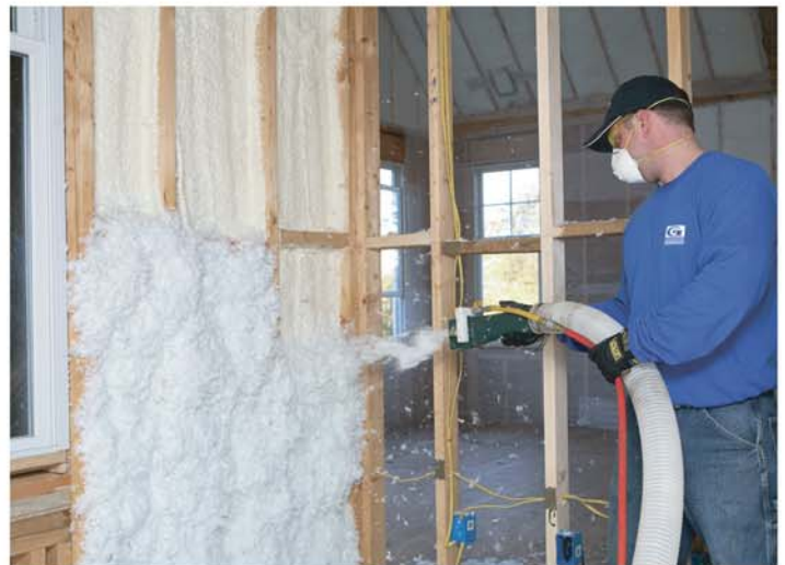
Application of UltraFit DS®/Asure R® loose-fill fiberglass insulation with ATS.
