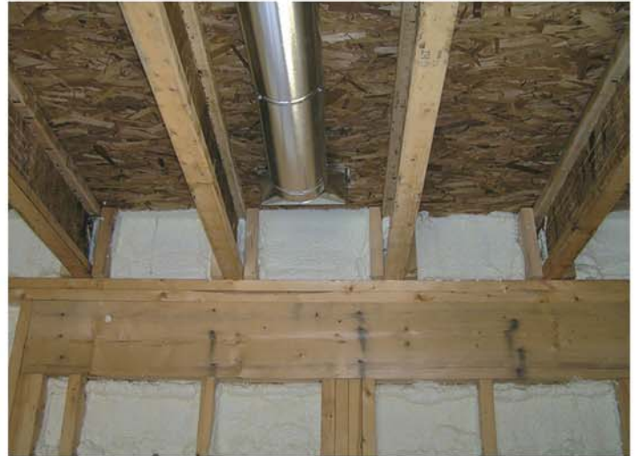
Application of closed-cell foam to joist ends and band boards.
