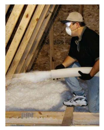
Attic Guard PLUS® is the perfect way to Insulate any attic space; whether it's new construction or retrofit.
